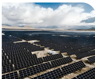
Solar power plant
